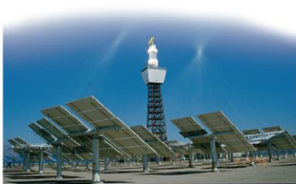
Solar power tower
